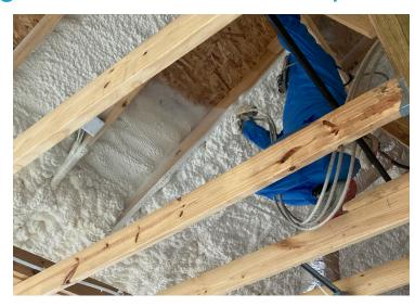
ENERTITE® X is a open-cell SPF insulation formulated for compliance with attic and crawlspace applications without the need of ignition barrier coatings. Simplify your open-cell SPF use in attic applications with BASF's Appendix X chemistry solution. ENERTITE X is ideal for insulation and air sealing applications in residential and commercial construction.
