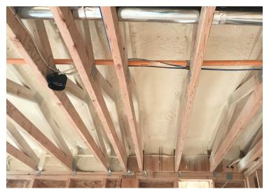
WALLTITE<sup>®</sup> Max is a lower-density, HFO-based closed-cell SPF insulation formulated for high-yield application performance while meeting GREENGUARD Gold standards and other robust requirements. It is ideal for insulation and air sealing applications in residential and commercial construction. WALLTITE Max provides contractors with improved yield, consistent thermal values, and superior application performance.
