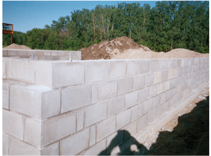
Basement Foundation Bare
