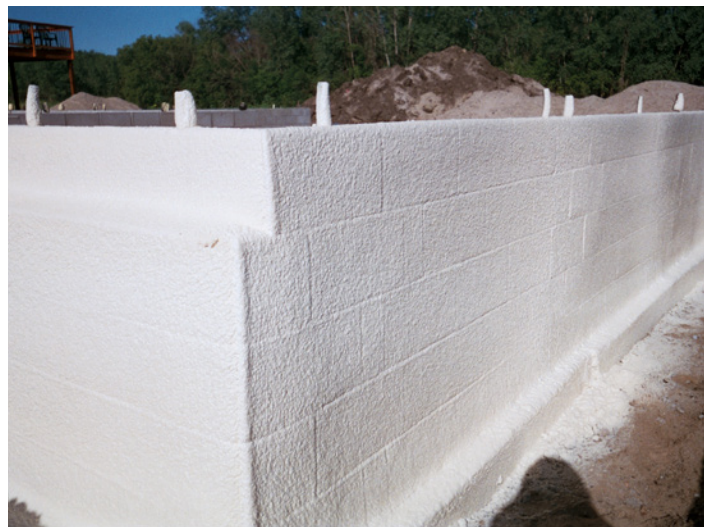
Foundation Spray Foam Insulation Applied
