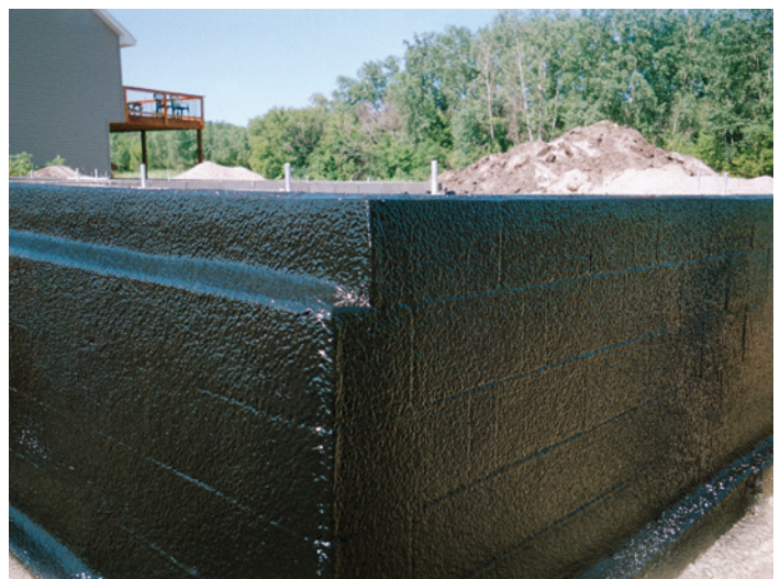
Waterproof Membrane (Polyurea 5 ) Applied
