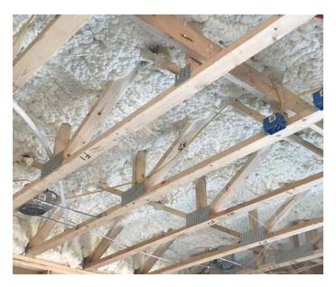
ENERTITE<sup>®</sup> Max is a low-density open-cell SPF insulation, formulated for high-yield application performance while meeting GREENGUARD Gold standards. It is ideal for insulation and air sealing applications in residential and commercial construction. ENERTITE Max provides contractors with improved yield, consistent thermal values, and superior overhead application performance.
